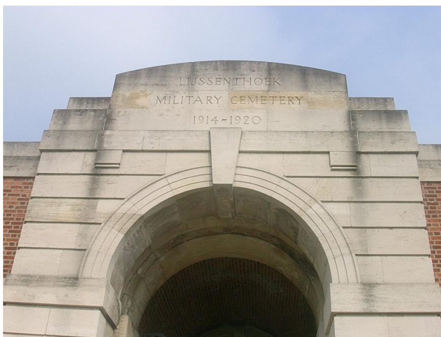
(Photo courtesy of International Wargraves Photography Project)
